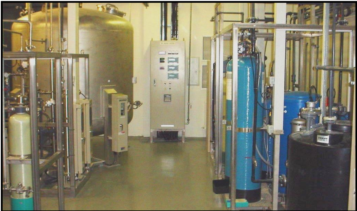
Purified Water Room
