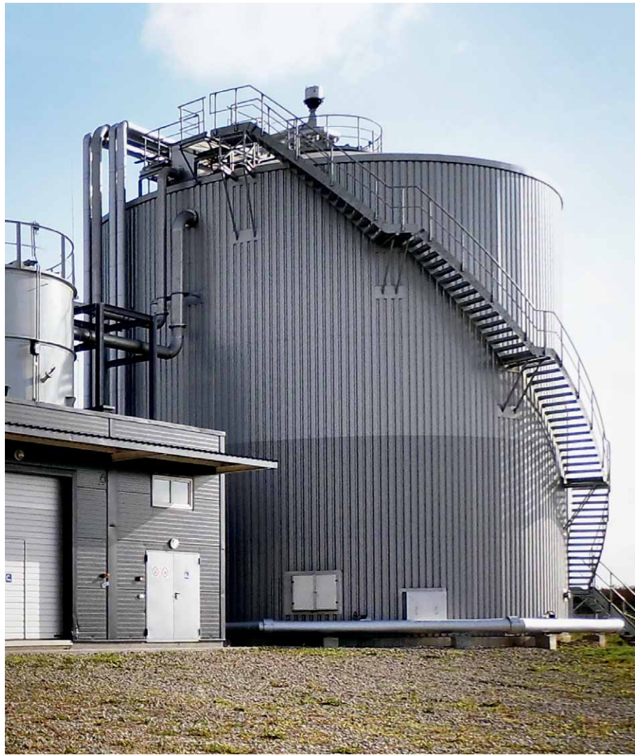
ANAFIT®.CS methane reactor with degassing stage and attached operational building for a HAGER + ELSÄSSER customer in Egypt.
