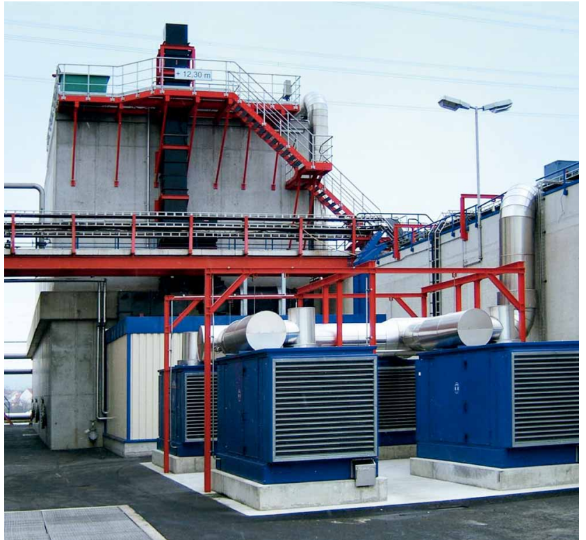
High load floating bed process BIOFIT®.H used in the BIOFIT®.Oxyd 2 process
