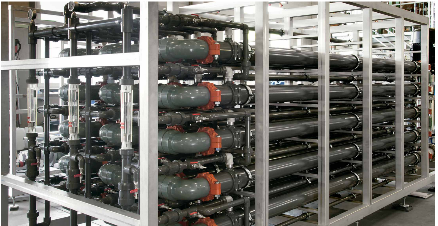
High pressure membrane stack for ZLD.eco 2
