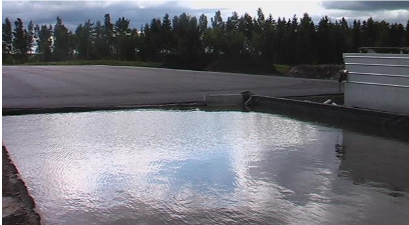
Mercury-containing wastewater in storage pond
