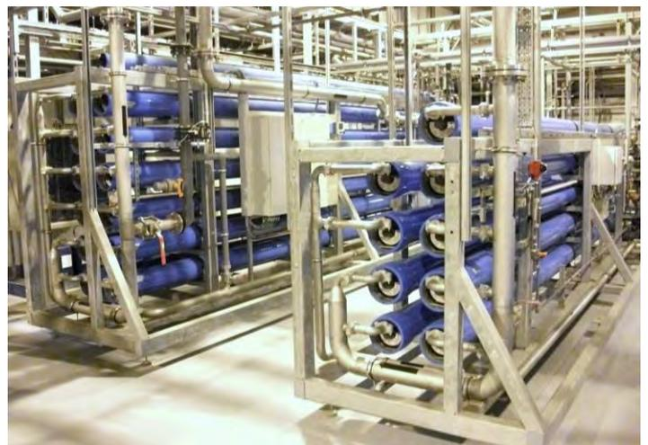
The product water from the twin-pass reverse osmosis system is then finally treated in two regenerable mixed bed deionisation polishers before flowing to a Deionised Water Storage tank designed to enable high flow rate and volume supplies at times of critical need.
