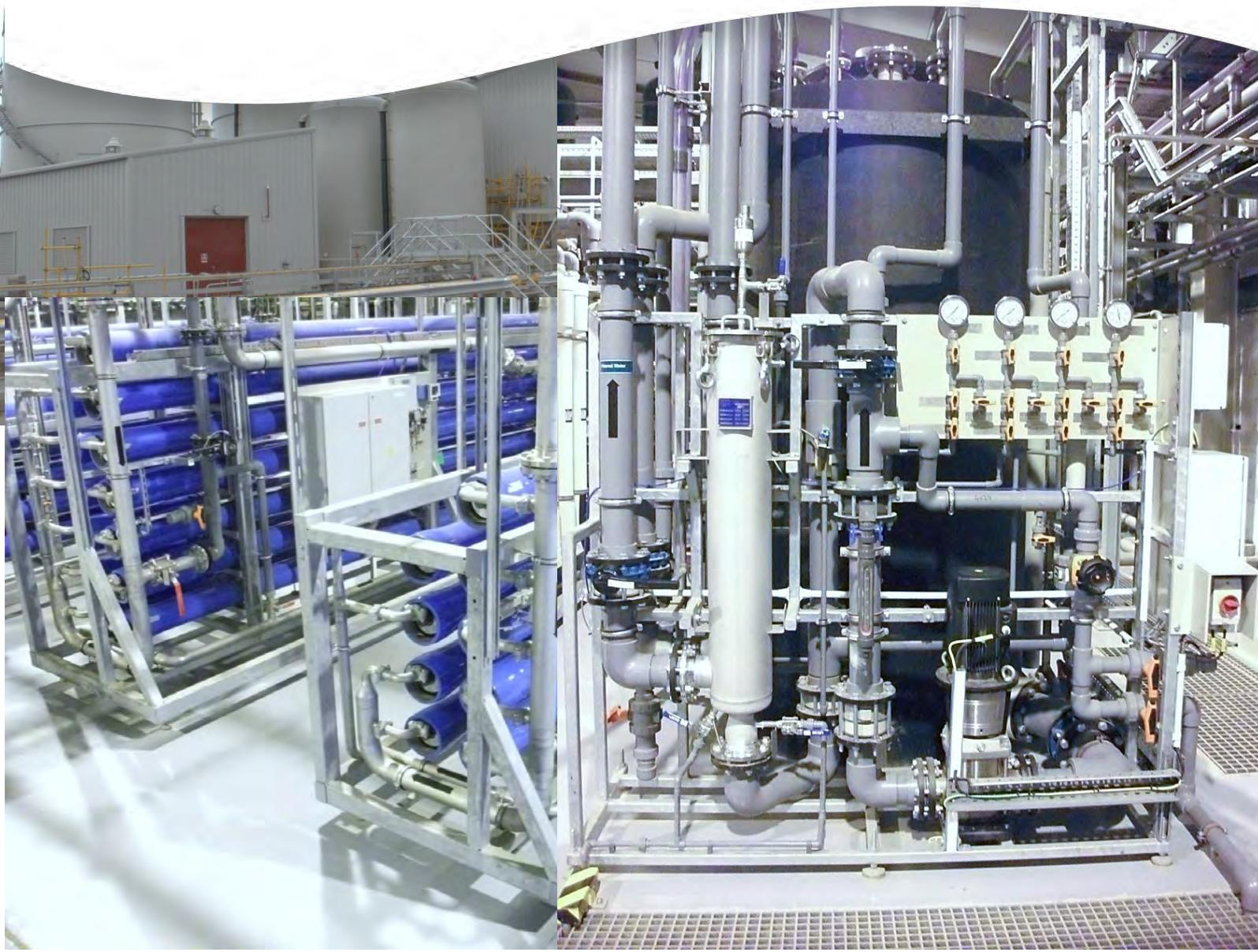
The recently built power station at Pembroke in South Wales is, at 2,160MW, the largest combined cycle gas turbine (CCGT) power plant in the UK. It was recently built for RWE npower by Alstom Power Systems. Hager + Elsässer was contracted by Alstom to supply the process water system to feed the gas turbines.
