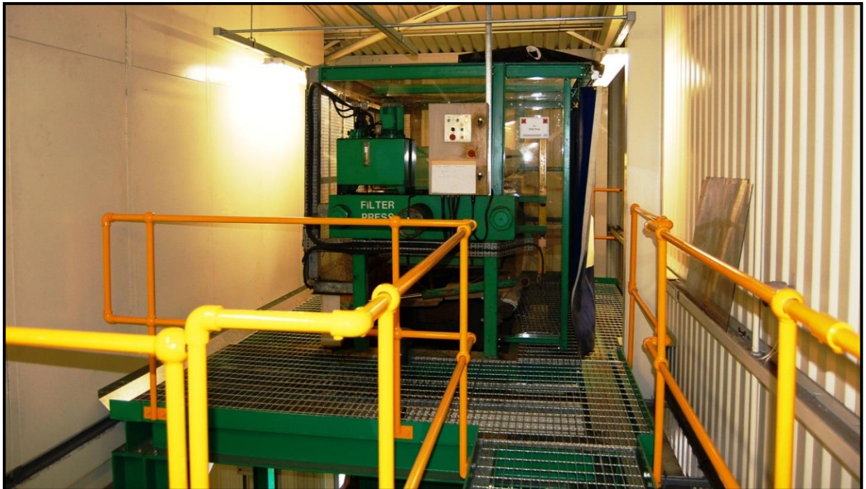
Fully Automatic Filter Press for Sludge Dewatering
