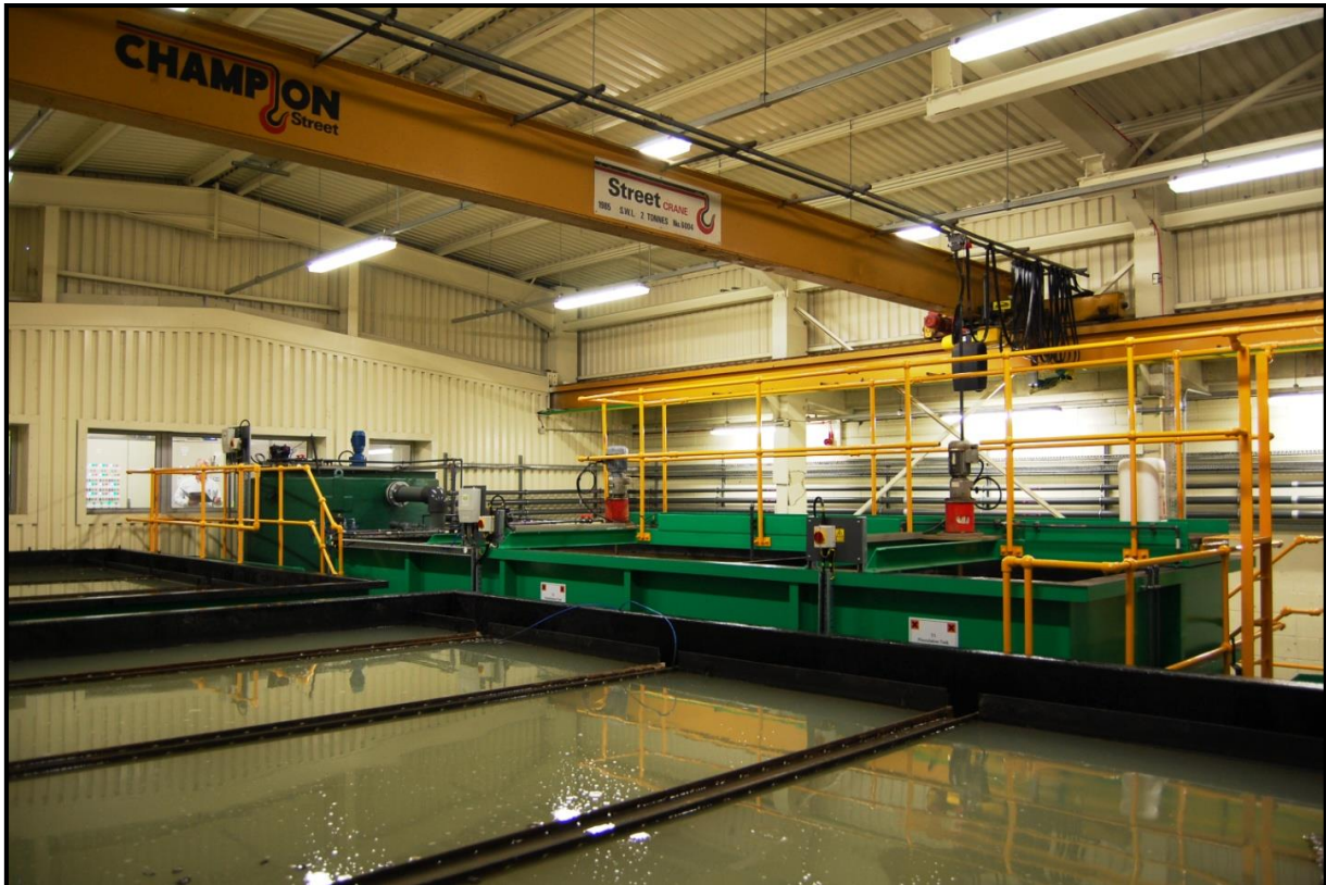
Treatment and Settlement Tanks
