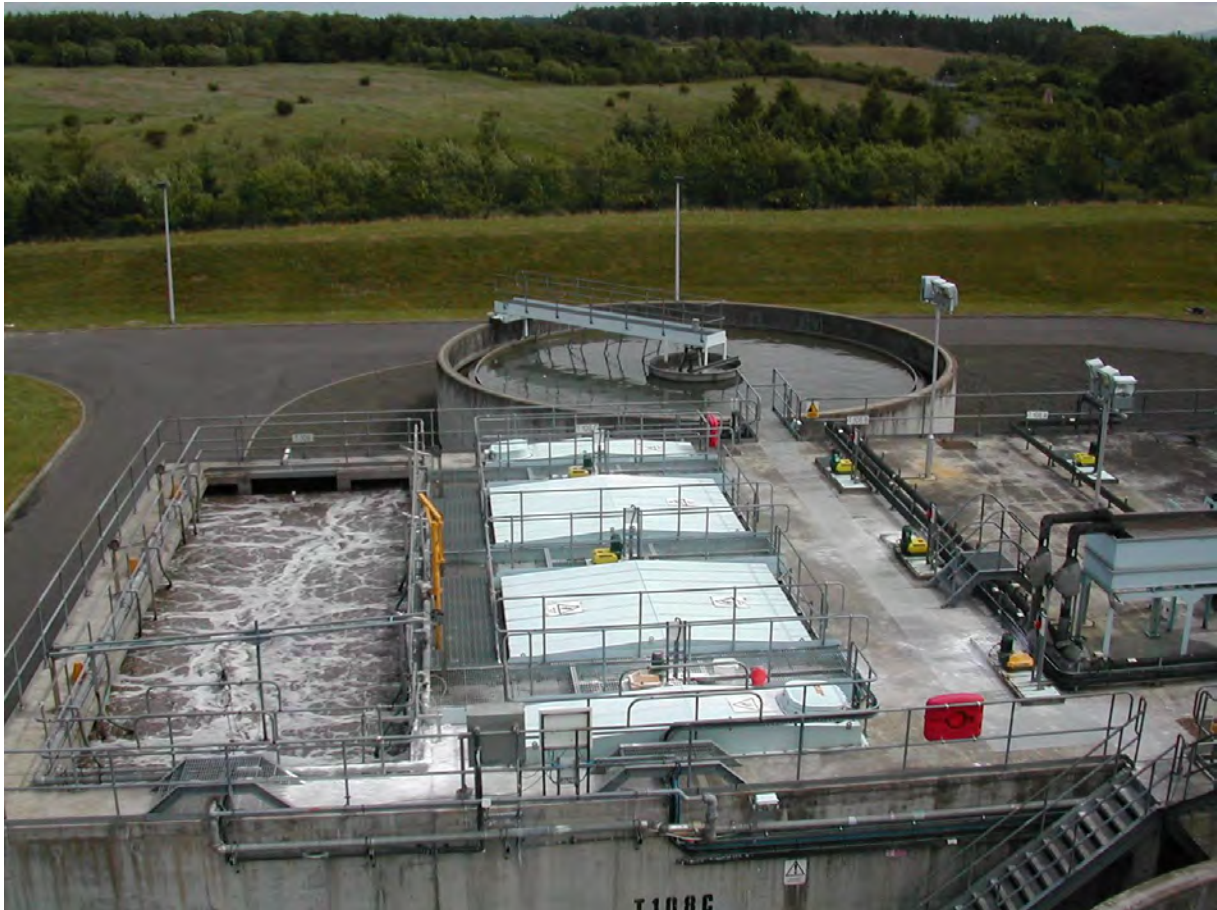
View of biological treatment outside the main plant building
