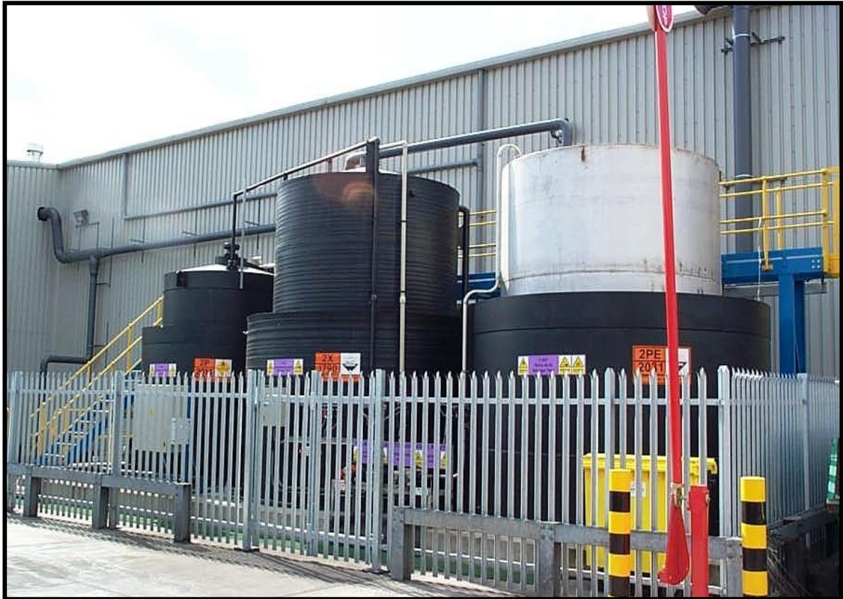
Bulk Pickling Chemicals Storage Facility
