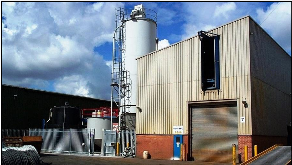
Main Effluent Treatment Plant Building
