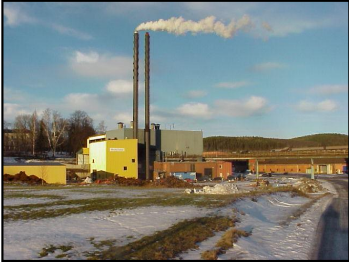
Hofors Energy AB, production facility within Ovako Industrial Park
